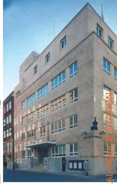
The design treatment of the exterior facade with the refurbishment of external Portland stone, Travertine marble and Granite stone has greatly enhanced the existing buildings features and emphasised its contemporary look. The areas of works included the demolition and clearance of all internal walls, ceilings, floor finishes throughout the building and significant reconstruction.
